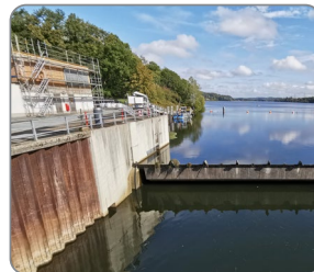
Hydropower plant Kemnade (DE)
