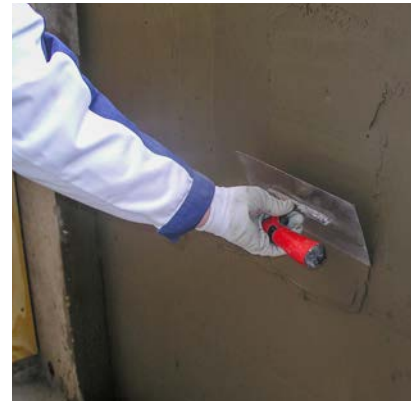
Application of BPA-CEMDicht 3 in 1 by troweling.
