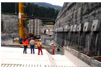
Tunnel Küblis | Switzerland
