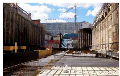
Train Station S21 Stuttgart | Germany
