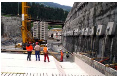
Tunnel Küblis | Switzerland
