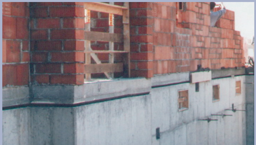
Figure 2: Stripped and finished horizontal joint
