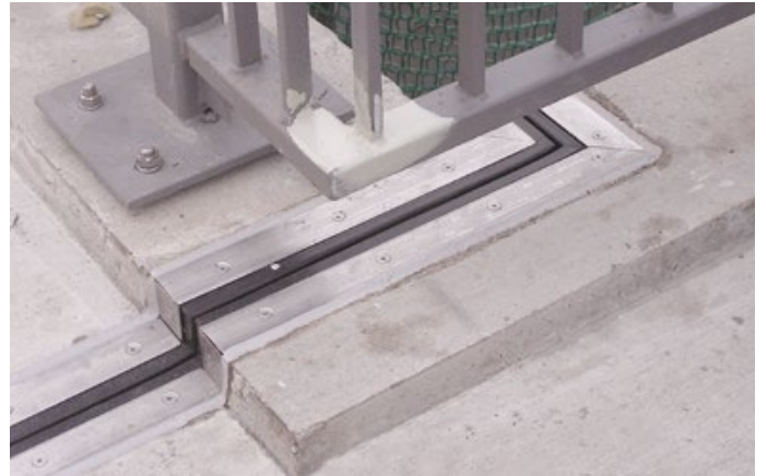
Refurbishment pedestrian bridge, Eilenburg, Germany
