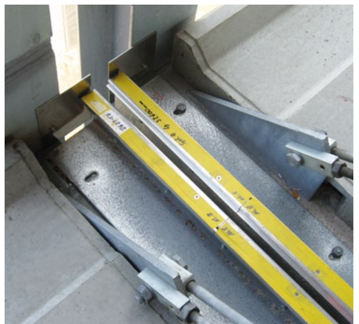
Parking garage Weiterstadt, Germany – FP 90
