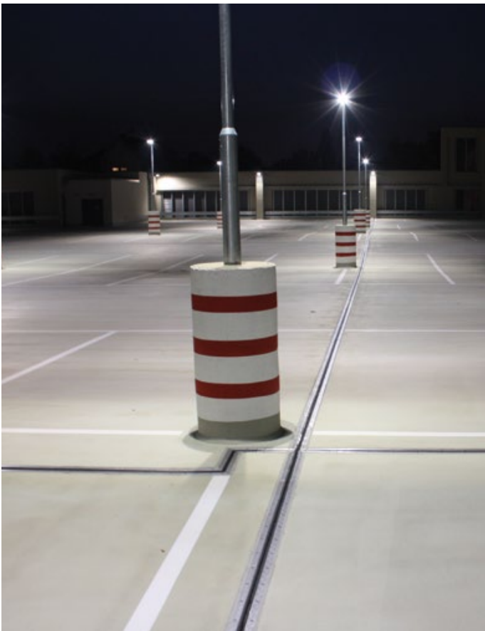
Parking deck shopping mall Dresden, Germany
