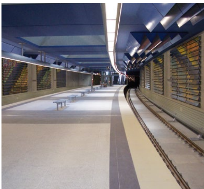
Hamburg airport, underground
