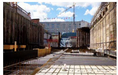
Train Station S21 Stuttgart | Germany
