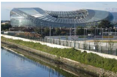
Aviva Stadium Dublin | Ireland
