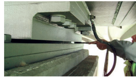
Installation of a fixed restraint device
