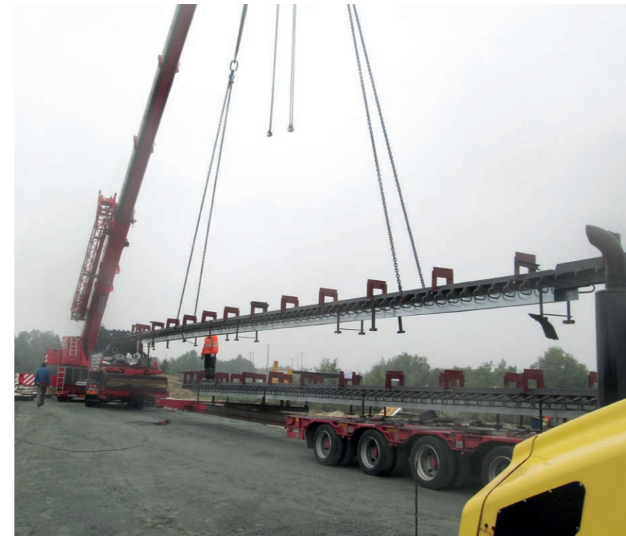
Handling and positioning of expansion joints with multiple steel profiles
