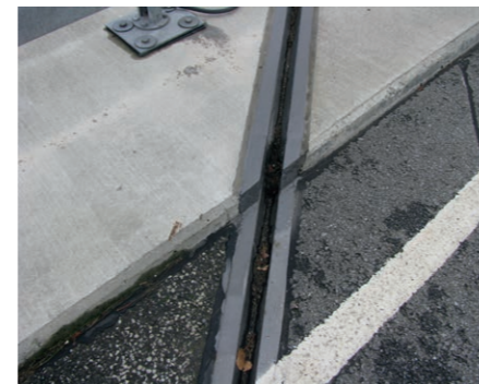
Flush-mounted steel profile in the walkway
