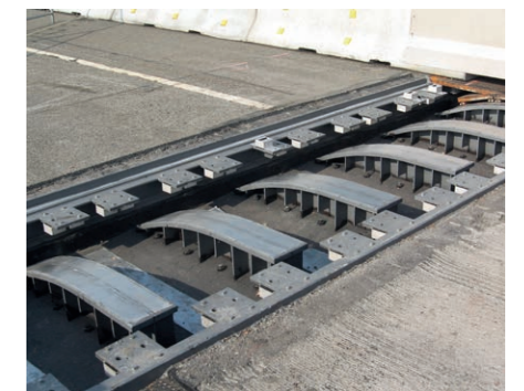
Roller shutter joint during installation
